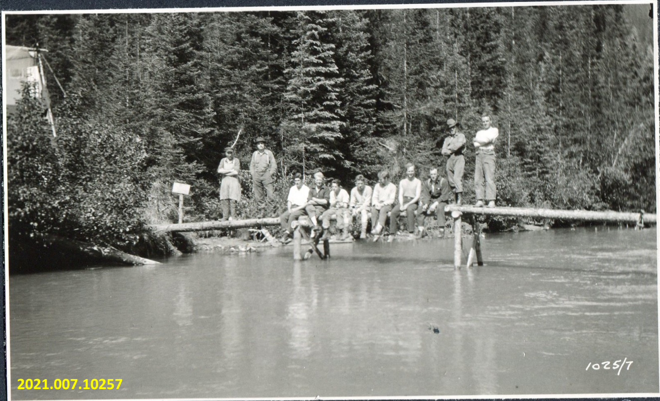
North Fork Horsefly River at Forks. Bridge built by Cruising Party. Barr. 1923.
